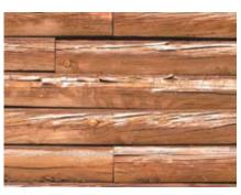
"Alligator Effect" due to weathering of unprotected surface.
