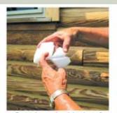
Cut triangular blocks of EPS or polyethylene foam.
