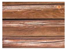
Checking and weathering of logs due to lack of maintenenace.
