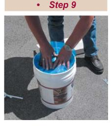
Replace the plastic liner over the surface of the sealant.
