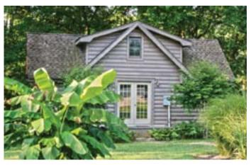
The cabin was built from a custom design, using Honest Abe's 8" x 8" D-Log profile, offering exceptional energy efficiency. It also features the company's Heavy Timber Roof and Ceiling Systems, which utilized large exposed beams for its structure. The family chose to use Lifeline Ultra-2 in Driftwood by Perma-Chink Systems for the stain, providing a washed and naturally weathered look to blend into the farm and river surroundings.
