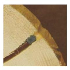
When initially applied 3/8" thick in a check the Check Mate 2 bonds to the sides of the check. As the check opens, the Check Mate 2 stretches to maintain a water-tight seal. The only role the Backer Rod plays is to maintain a Check Mate 2 thickness of 3/8" during the application.
