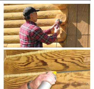
The decision was also made to apply the finish after the lightly textured *Energy Seal*® had been applied and allowed to cure. Using this method, the sealed joints will blend in nicely with the overall appearance of the surface.
