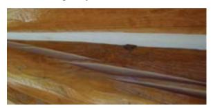
Check-Mate 2 applied to upward facing check
