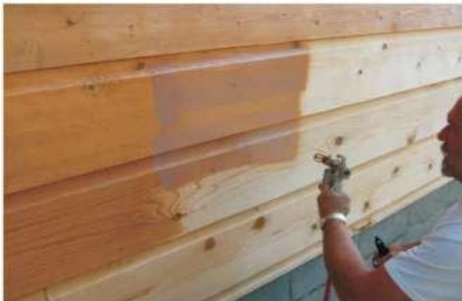
Spray apply finish to a small area
