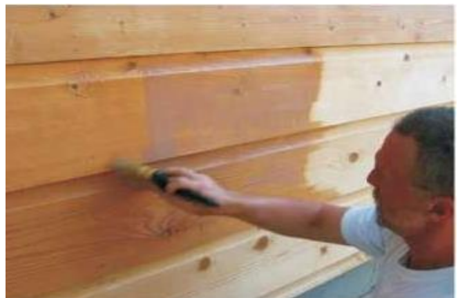
Back-brush finish to obtain a uniform film
