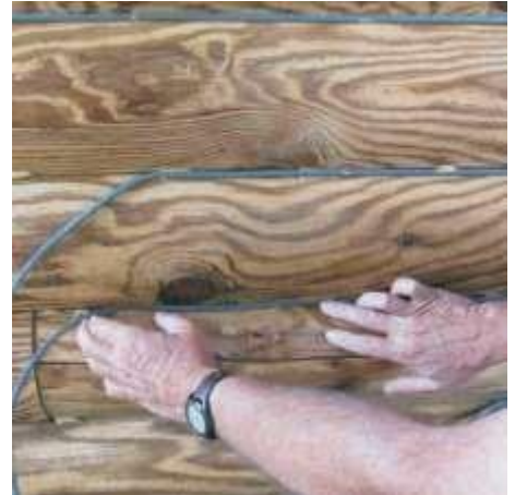
Attaching Backer Rod
